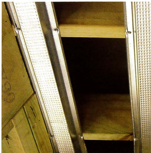
Direct fix to trusses
